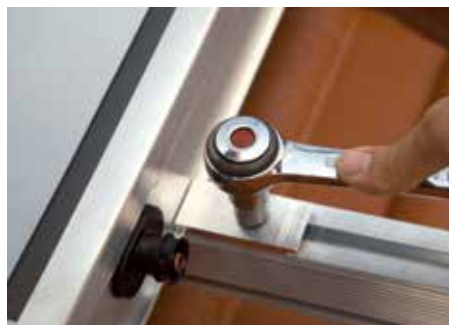
Fixing of collector to rail
